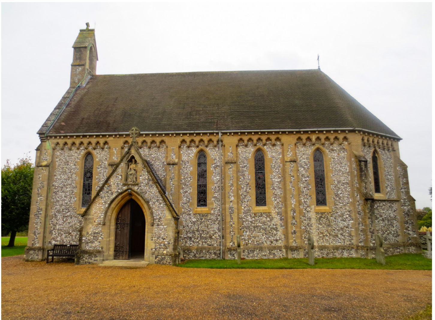
The exterior of St Edward the Confessor, Sutton Park, near Guildford
